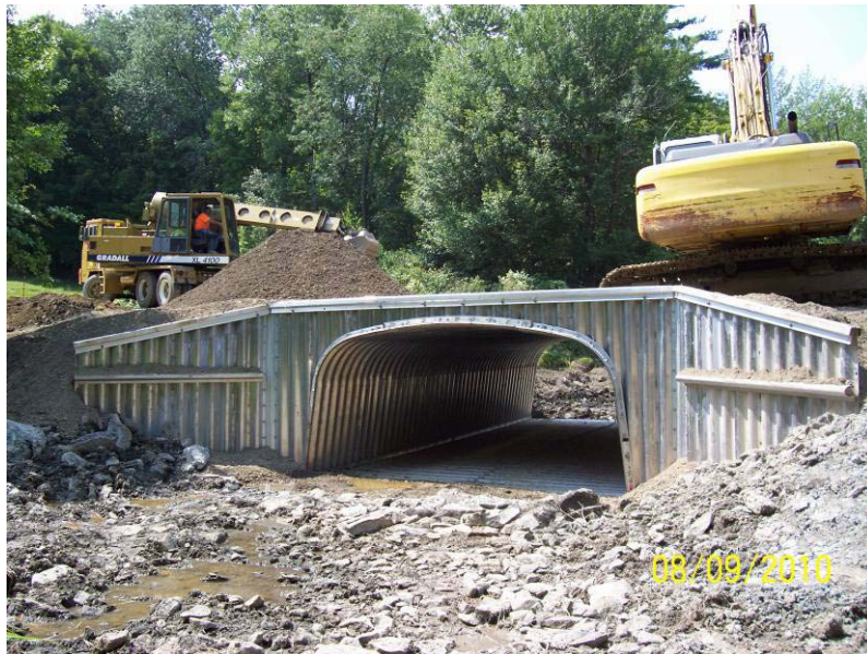
County Work Crews Replace Bridge on South Road in Grafton, August 2010
