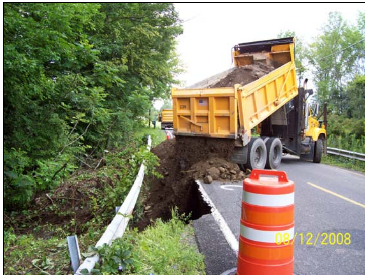
County crews repairing storm damage, August 2008
